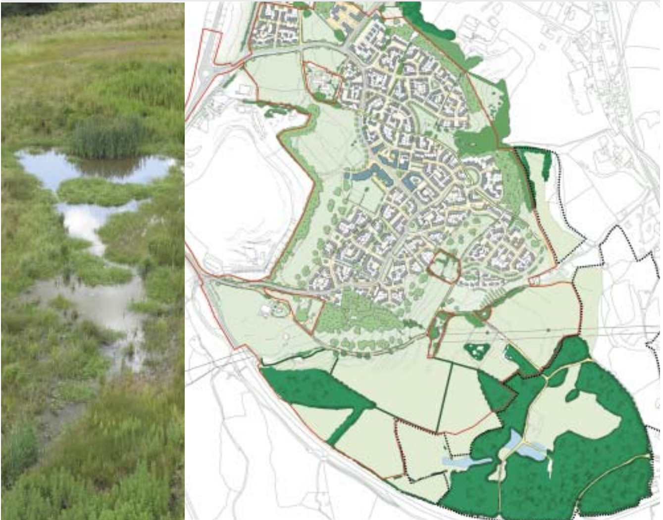
Maintenance costs for Lightmoor Village SUDS scheme are generated from residents' service charges.
