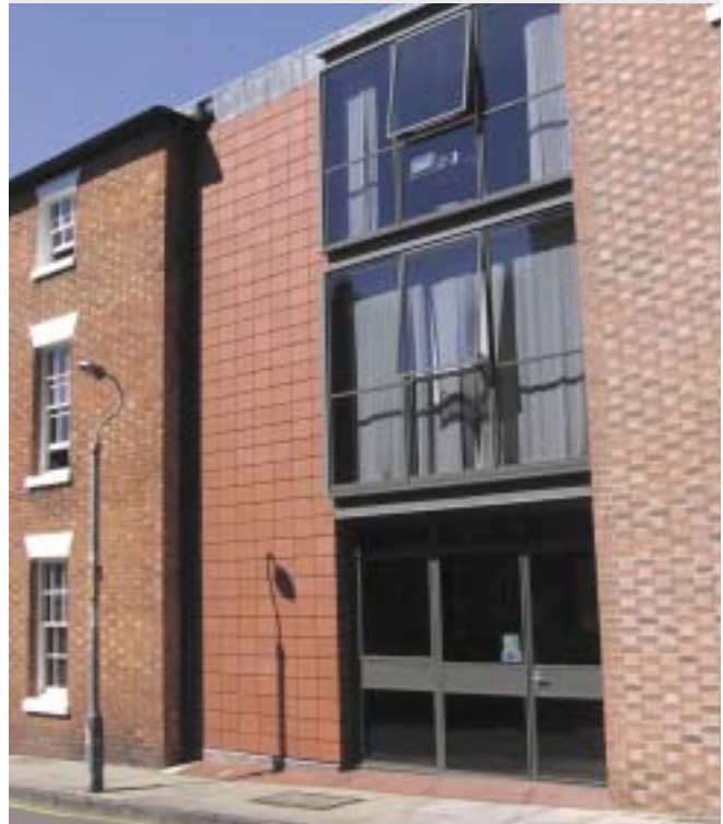
The Stratford-on-Avon District Design Guide has assisted in delivering contemporary schemes which respond to the characteristics of the area.
