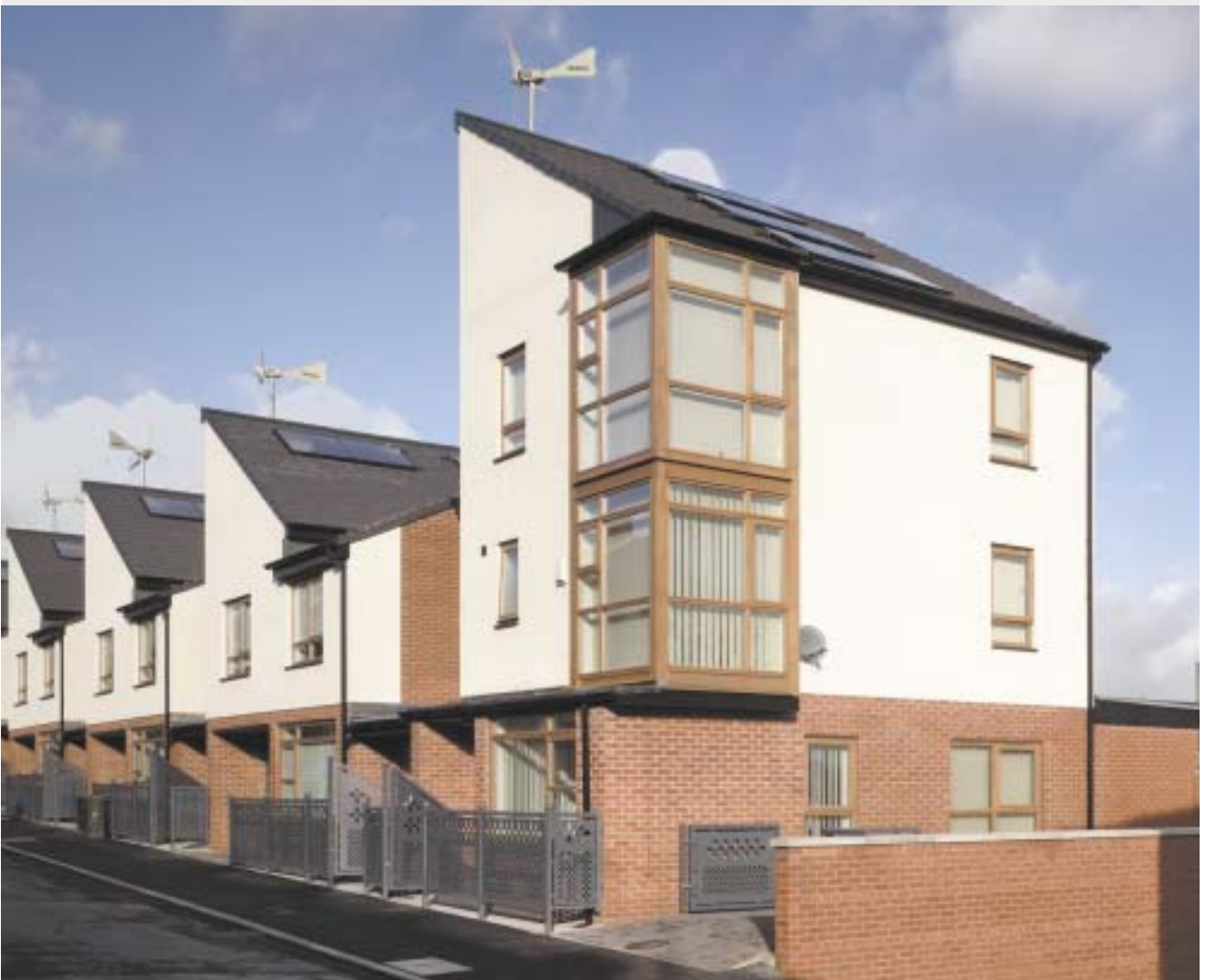
Terraces along Selwyn Street are orientated to avoid overshadowing in rear gardens and monopitched roofs are designed to face south east to maximise solar gain.
